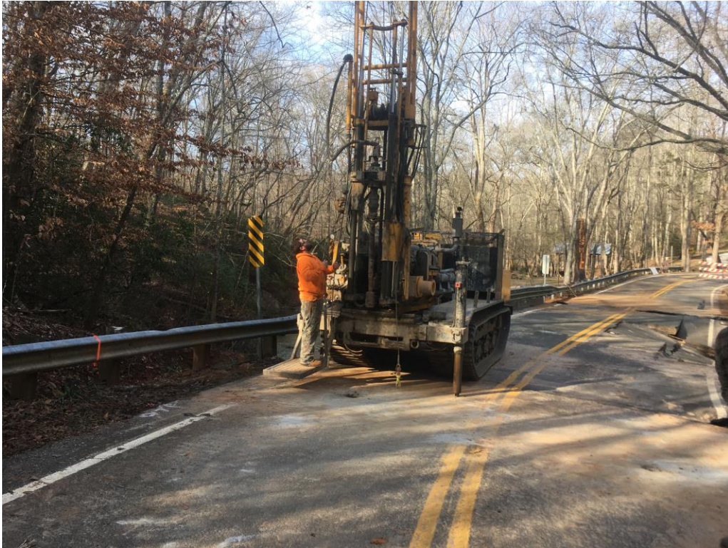
Photo 1: Drill Rig at Boring B-1
