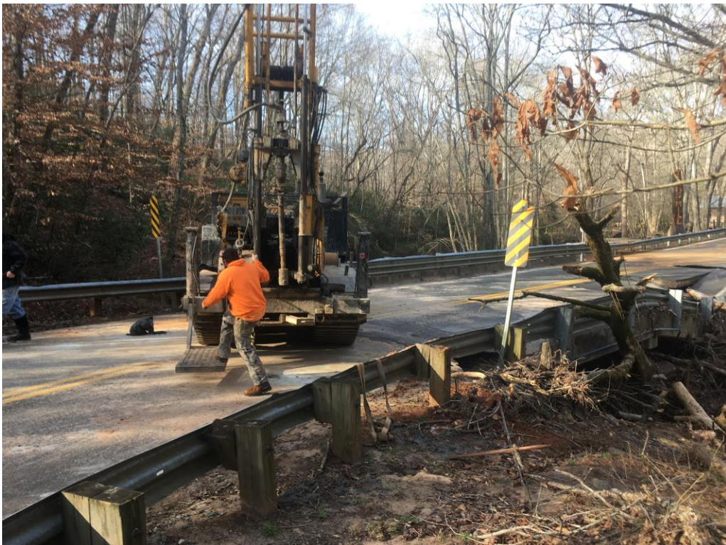
Photo 2: Drill Rig at Boring B-2
