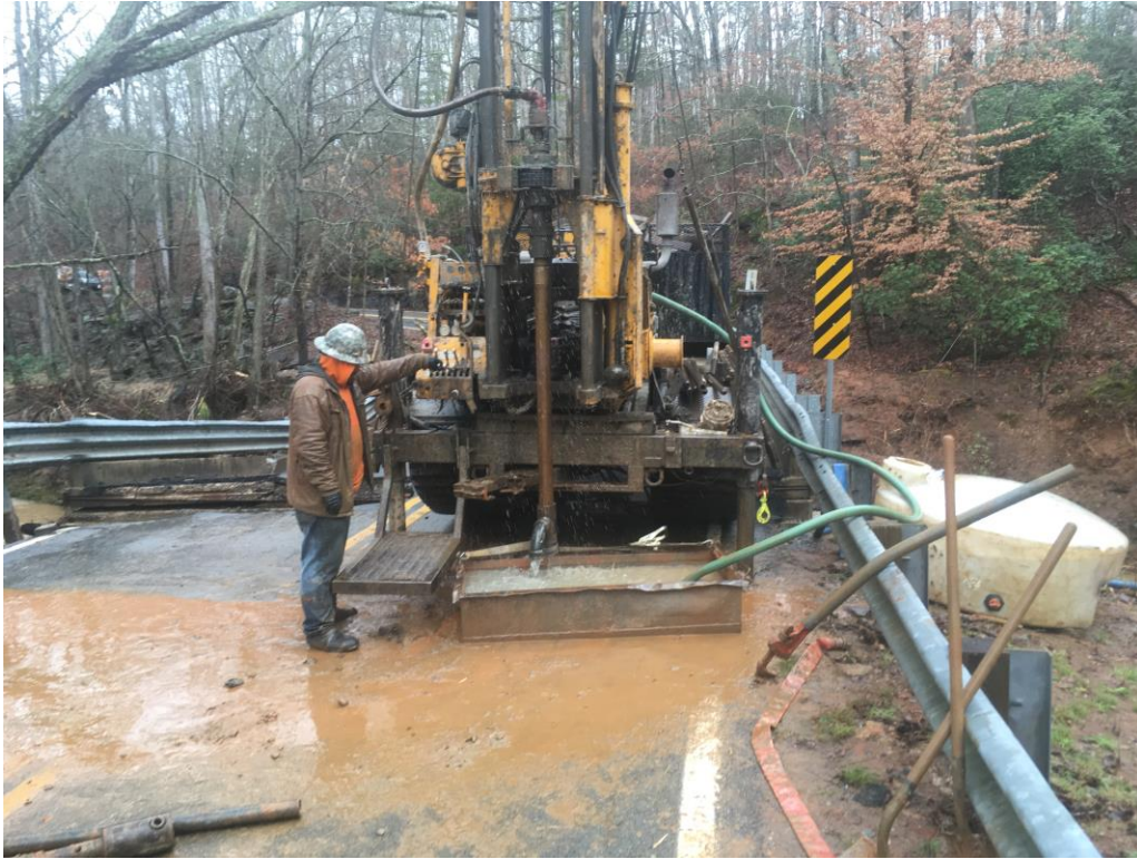
Photo 3: Drill Rig at Boring B-3
