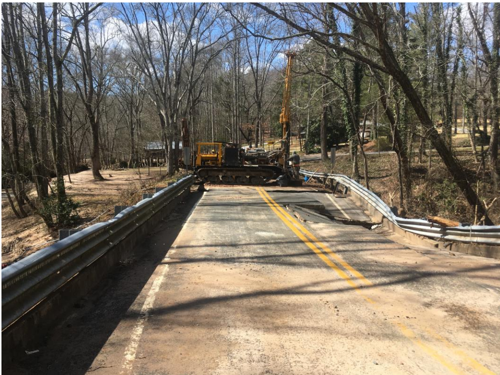
Photo 4: Drill Rig at Boring B-7
